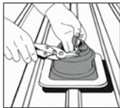
1. Adjust DEKTITE® to the pipe.
